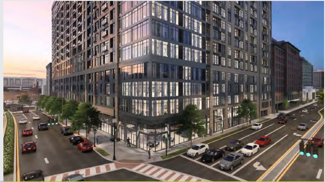
View of Washington Boulevard and Tresser Boulevard
